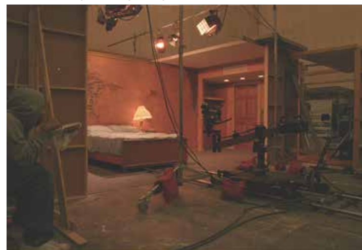
Motel Room: Art Director/ Construction Coordinator. Built on stage, this 360 set had several fly-walls for flexible shooting and lighting.
